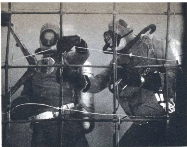
2 TORPEDO NET protects channel. Attached to cable are electrified wires which sound an alarm when cut.
